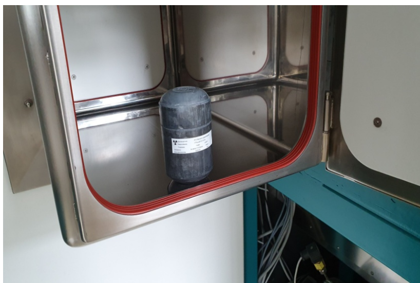
Figure 36 - Transfer of the container with the drug for quality control through a ventilated gateway
